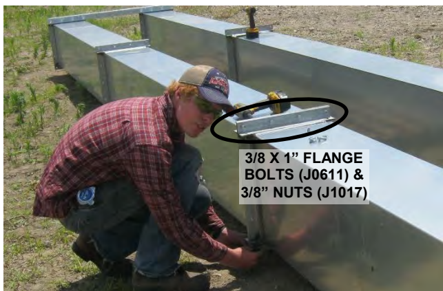
Image 3 – Bolting flanges of second leg together
