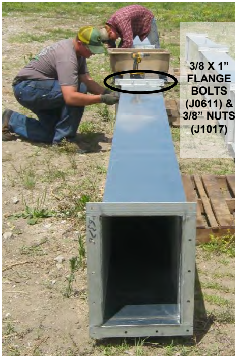
Image 1 – Positioning 10' trunking sections & bolting flanges
