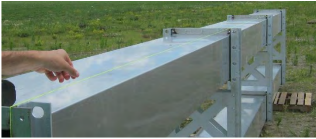
Images 14 & 15 – Checking alignment
