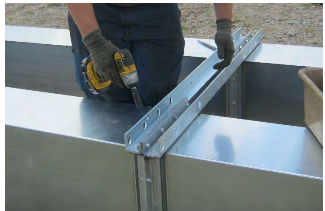
Image 4 – Bolting tie angles to flanges
