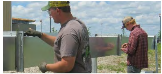
Image 6 – Bolting flanges together
