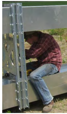
Images 7-10 – Attaching tie angles, squaring plates & alignment pins
