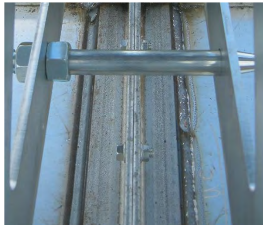
Images 11-13 – Attaching alignment pins
