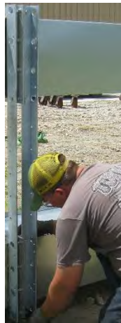
Images 7-10 – Attaching tie angles, squaring plates & alignment pins
